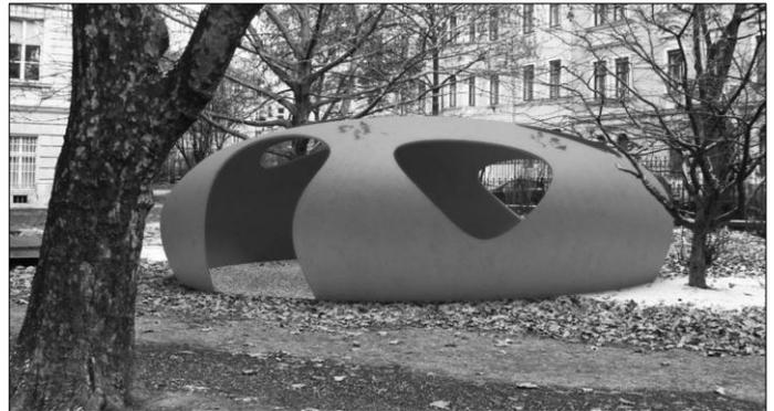
Figure 3. Prefabricated UHPC shell construction – student work by Stephanie Jordan, Nikolaus Pfusterschmied and Felix Zmölnig (TU Graz, 2012).
